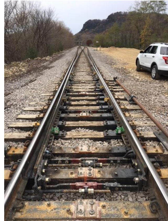
End of Two Main Trks Winona Jct. 60 mph #24 Equilateral
