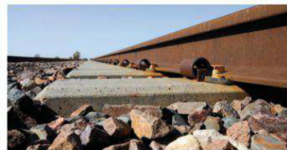
Concrete ties weigh as much as 750 pounds each and stabilize track with their weight and tight fastenings. TRAINS: Brian Schmidt
