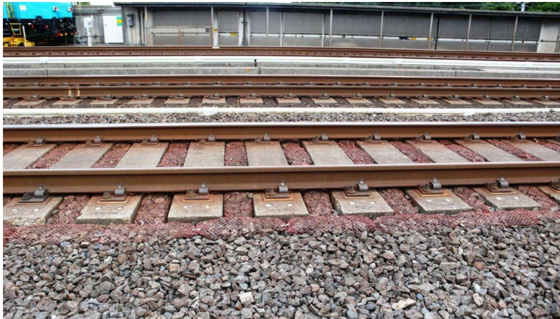
Figure 3.4: Ballast bags placed on the Japanese Shinkansen
