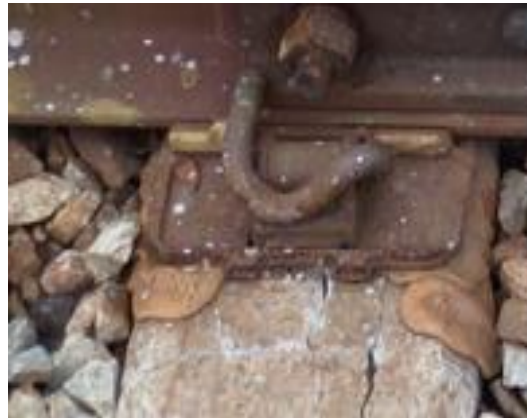
Rail Seat Epoxy Remediation
