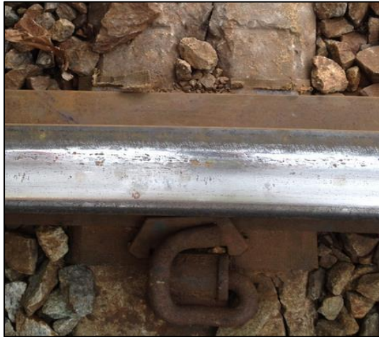
Broken/Worn Insulator
