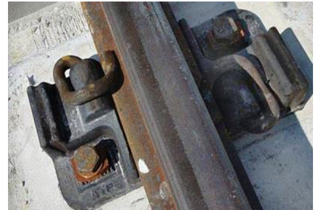
Direct Fixation Fastening System
